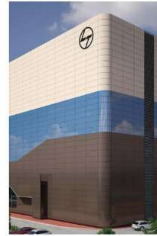
BEHIND L&T DATA CENTRE
