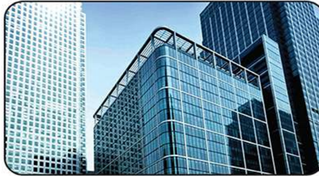
NEAR L&T DATA CENTER
