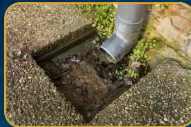
RAINWATER HARVESTING SYSTEM
